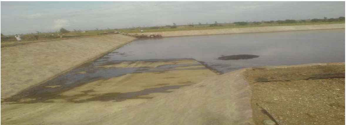
Construction of Impervious Spent wash Storage Lagoon
